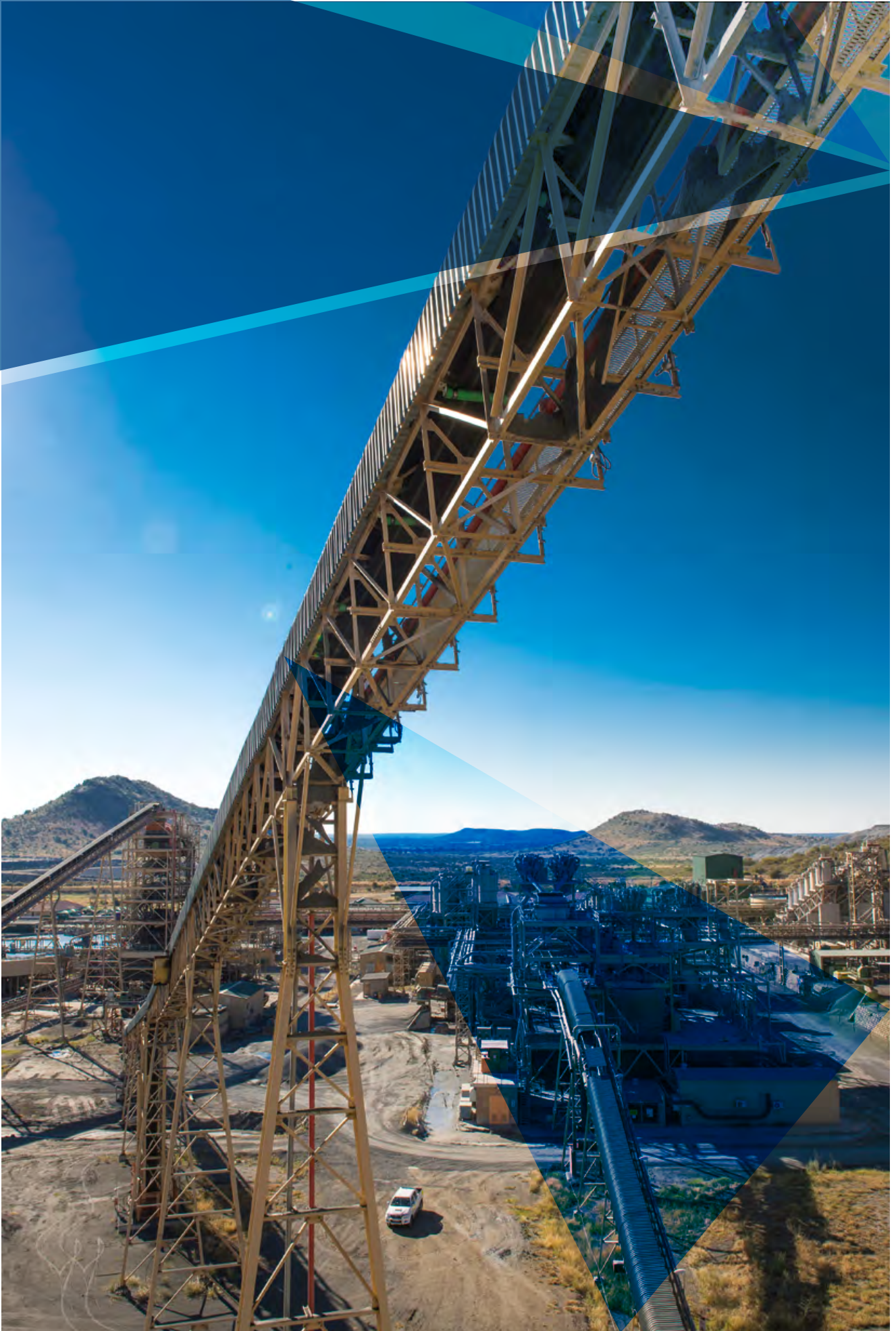
The concentrator plant at the Pilaesberg Platinum Mine.
