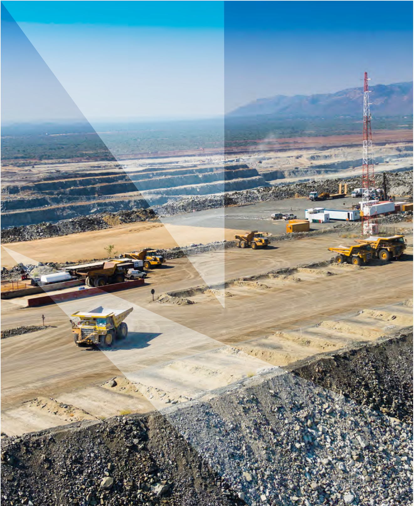
Birdseye view of Sedibelo's open cast Pilanesberg Platinum Mine.
